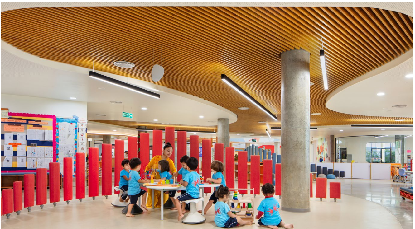
Image 17: Sound-absorbing ceiling, wall and free-standing panels can greatly minimize noise levels.
